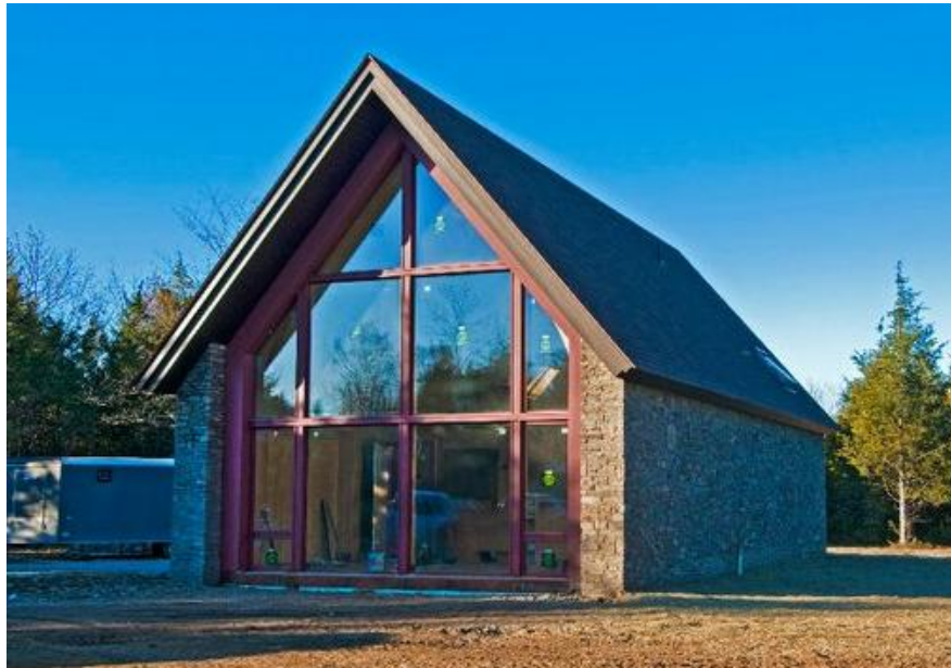
Figure 5. The Hudson Passive Project in Claverack, NY
