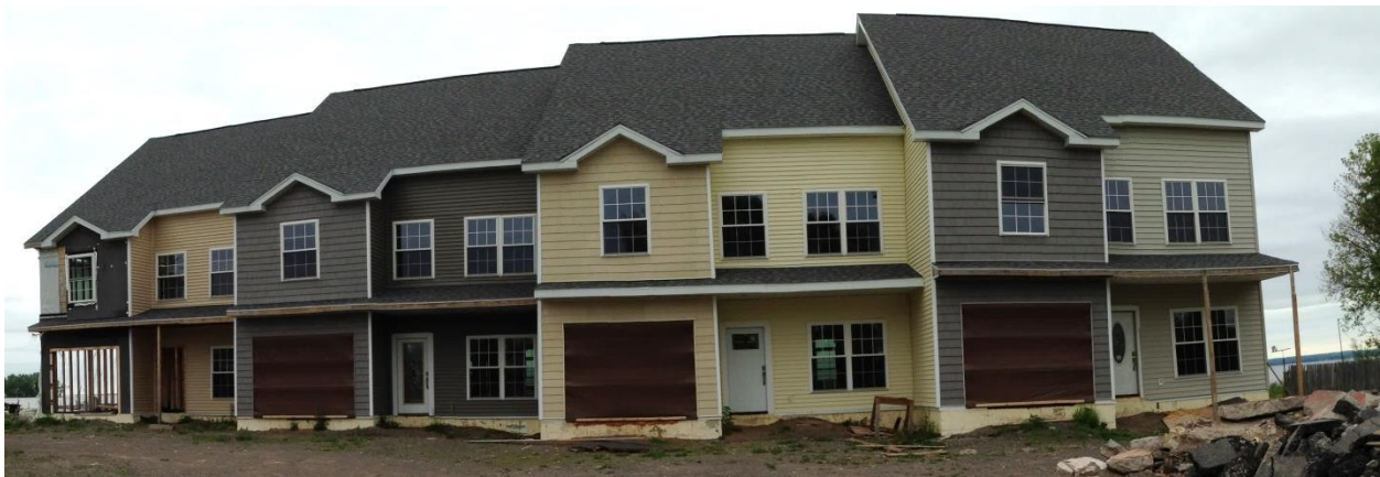
Figure 6. Weletok Townhomes Under Construction
