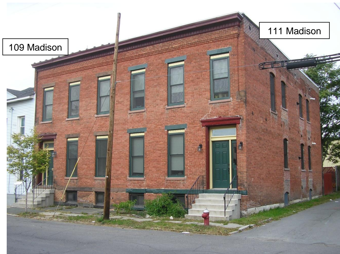
Figure 3. Photo of Two Buildings at Madison St (after renovation was complete)
