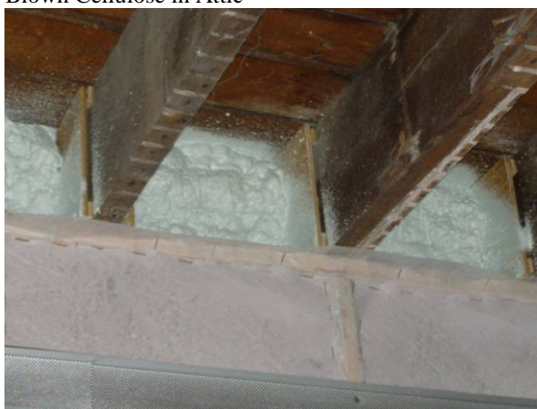
Closed Cell Spray Foam in Rim Joists
