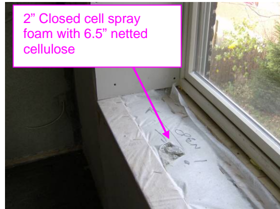
Rear Wall Detail at Window (drywall returns)
