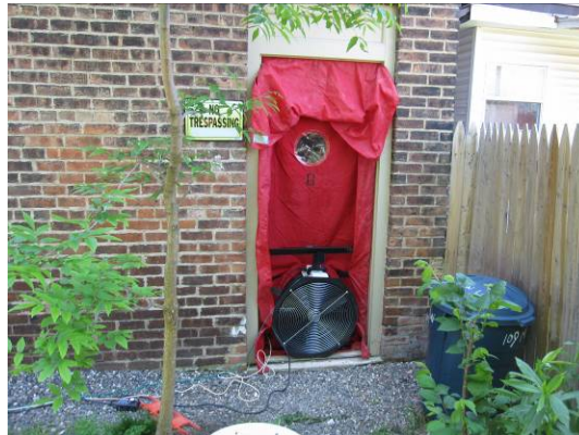
Fan door in old part of building (109 Madison St.)
