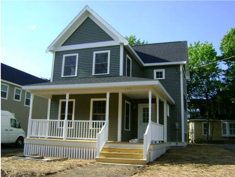
Figure 1. Photo of House
