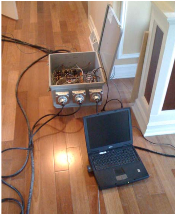
Setup for co-Heat Test
