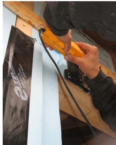
Tool used to cut out foam around the windows
