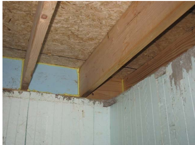
Foam Board Scraps used in Rim Joist
