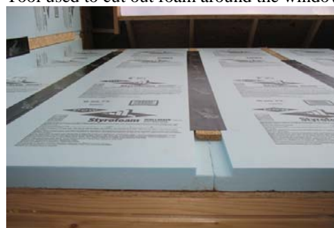
Furring strips with tape applied
