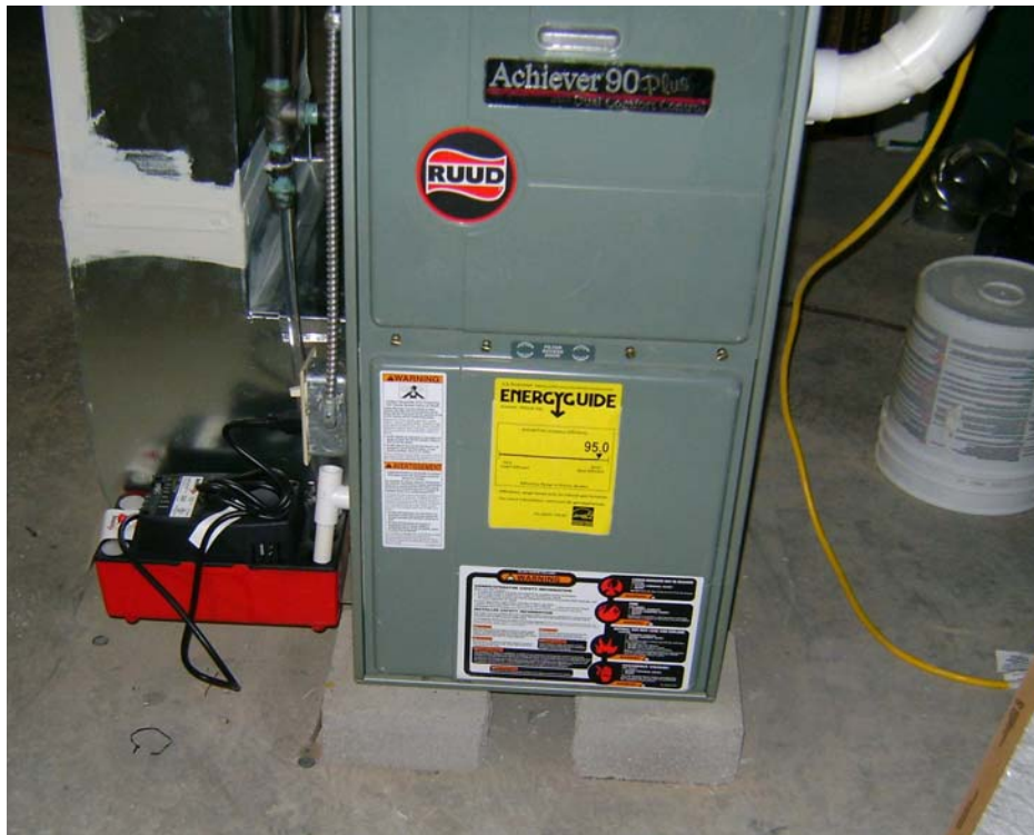
Figure 5. Two-Stage Gas Furnace
