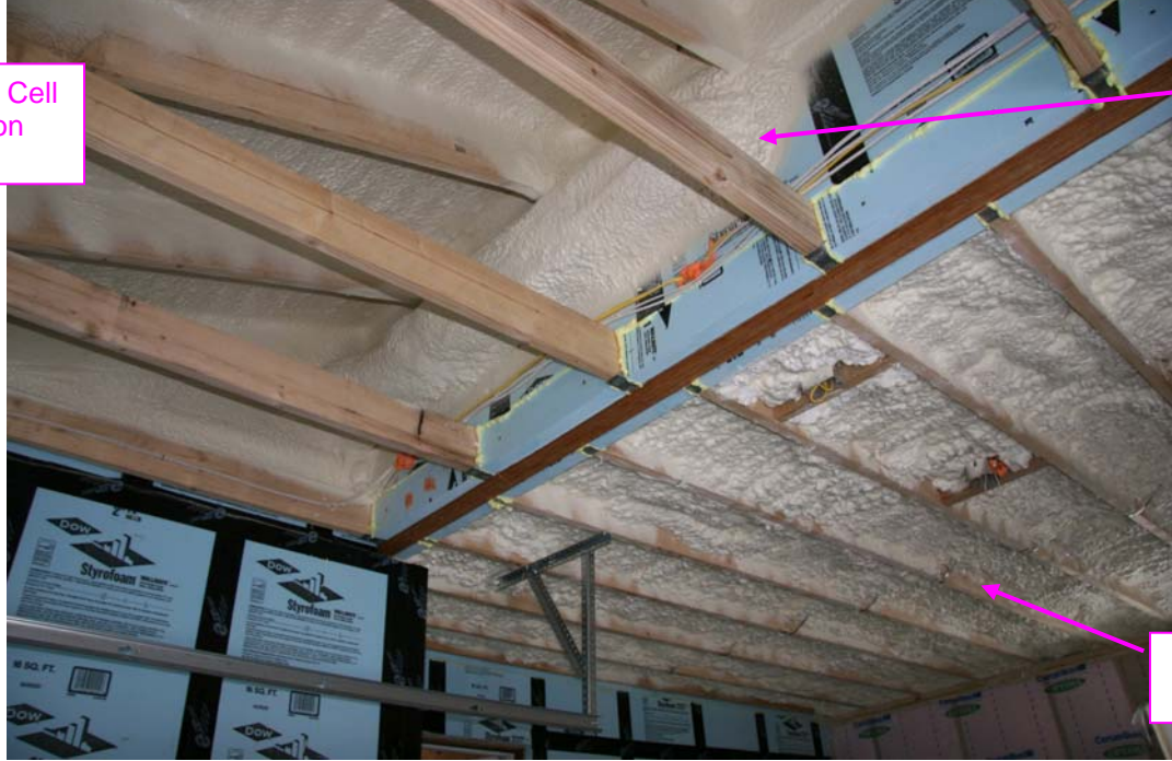
Figure 2. Insulation Shown Inside the Garage (rigid foam applied before drywall)
