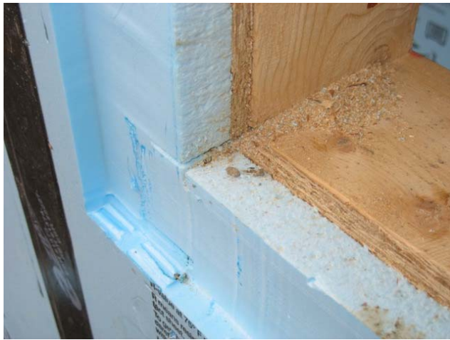
Foam cut back around the window
