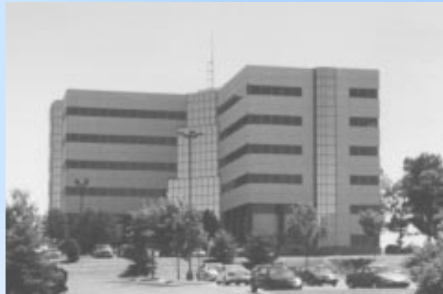
Middleton, WI Office Building
