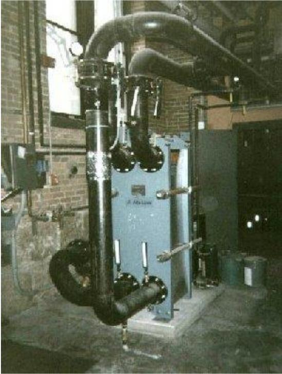
Figure 1. Plate Frame Heat Exchanger
