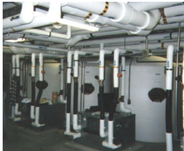
**Figure 5. Water Heating System Heat Pumps and Storage Tanks**
