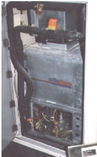
**Figure 4. Typical Single Room Heat Pump Unit**
