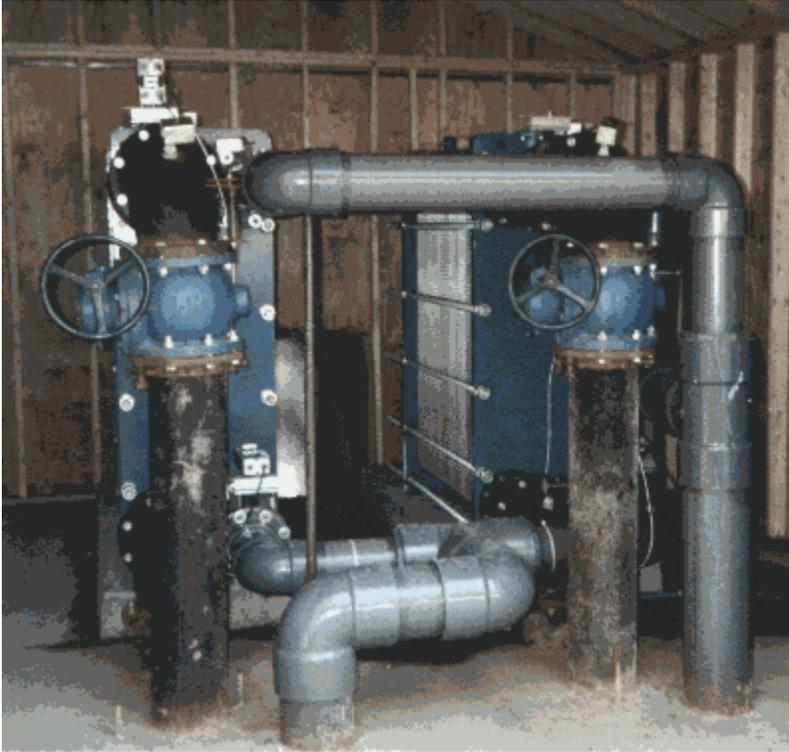
Figure 2. Plate Frame Heat Exchangers
