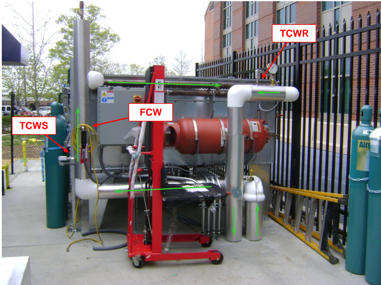
Figure 6. Locations of Cooling Module Temperature and Flow Sensors
