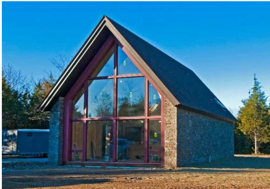
Figure 1. The Hudson Passive Project in Claverack, NY
